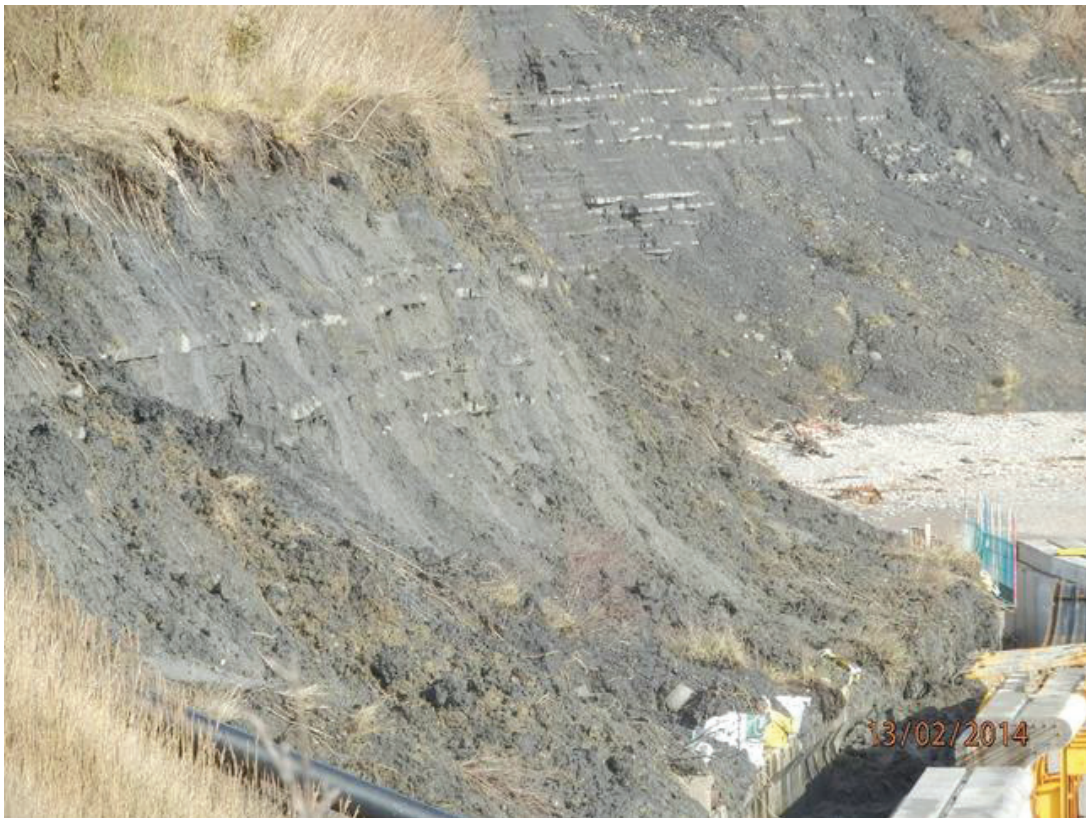
Figure 6 - Landslide area: Stable limestone marker beds visible
