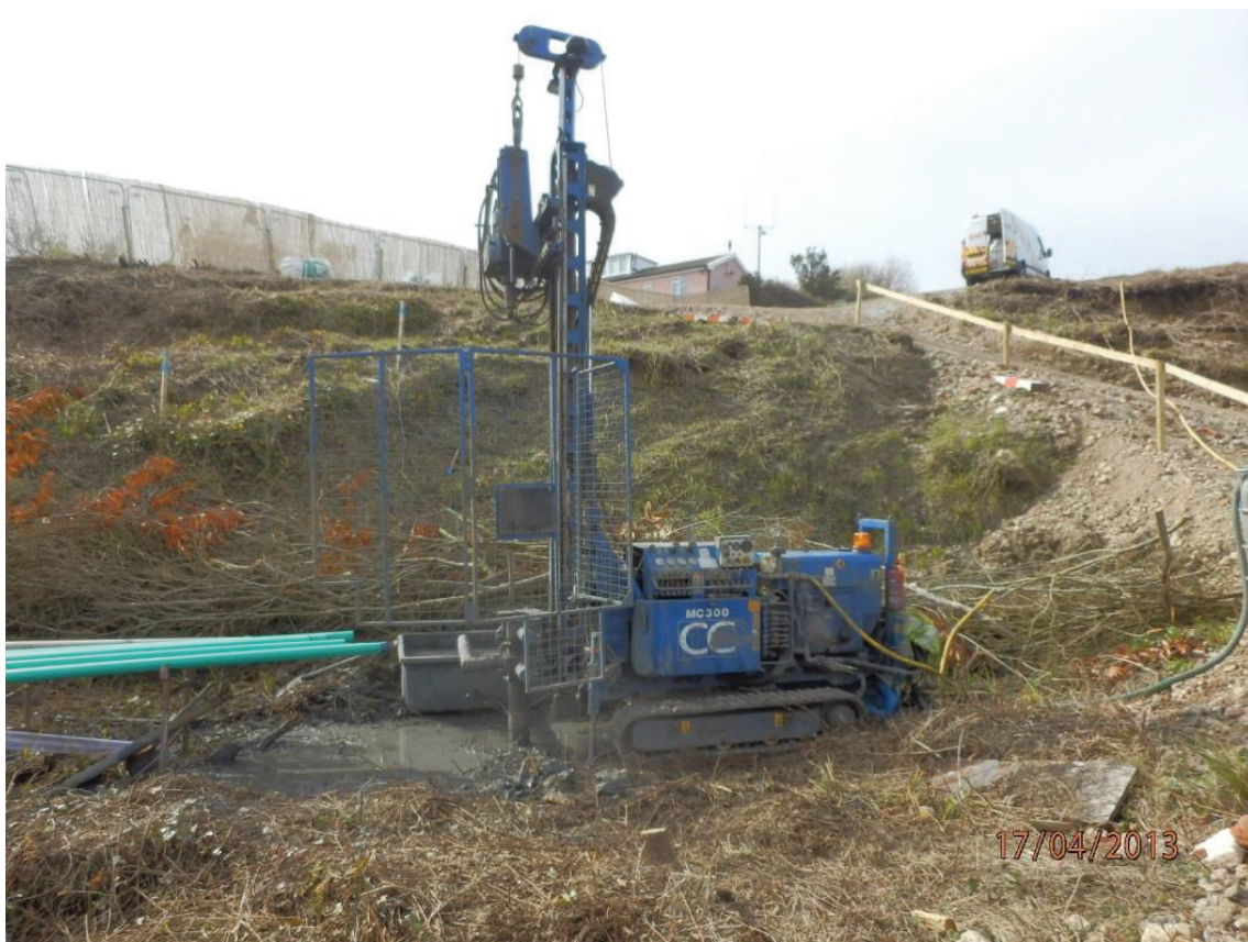
Figure 2 - SI drilling rig. Note landslide scars behind rig. The green tubes are grooved inclinometer tubes to be inserted and grouted into the bore hole
